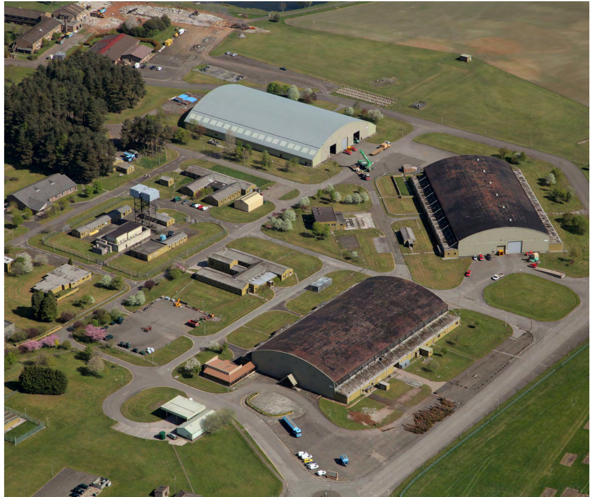
Figure 2.5.1 Former RAF Edzell Base hangars
