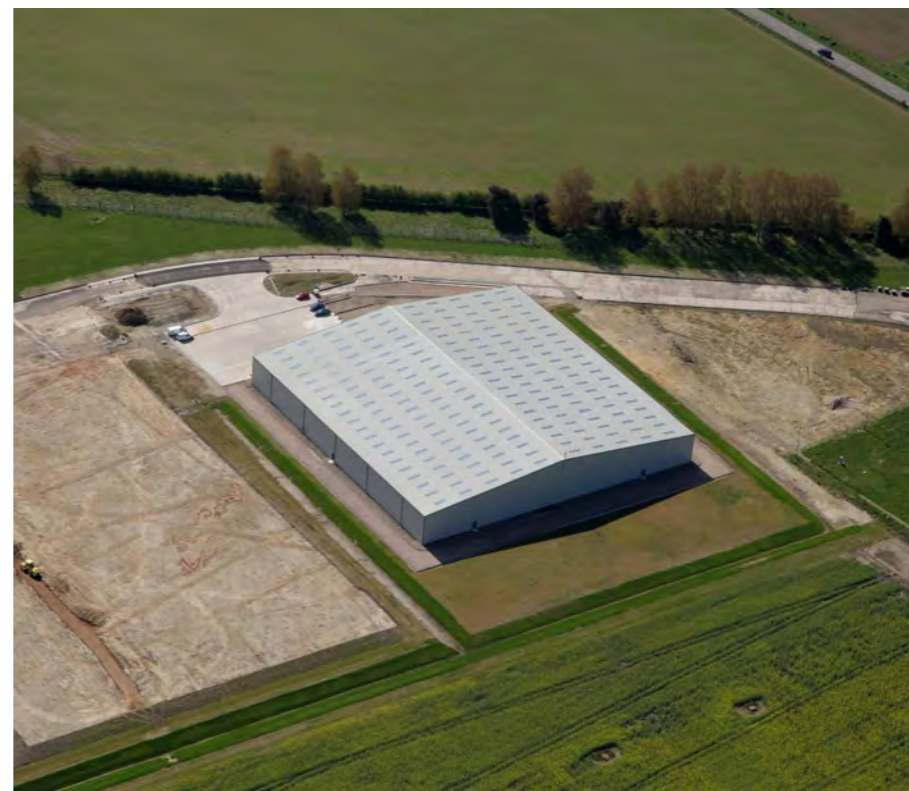
Figure 2.3.3 New Warehousing at the Edzell Business Base
