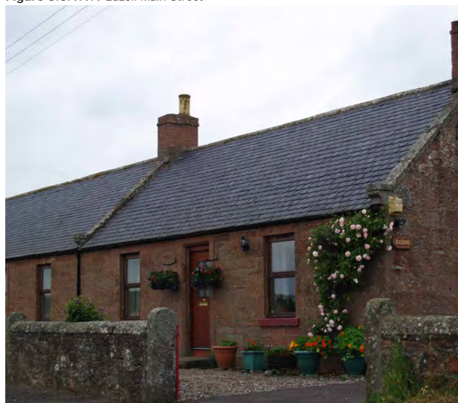
Figure 3.6.1.1.2 Edzell: Typical Vernacular Cottage
