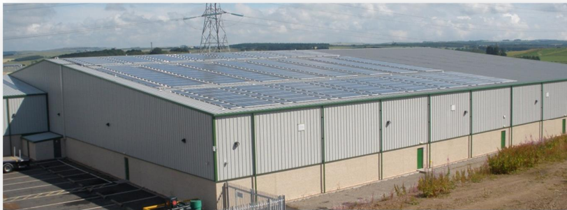
Figure 34 – Photo Voltaic panels sited on existing building at Midmill South Business Park
