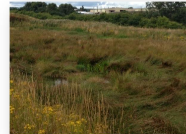
Figure 20 – Existing SUDS pond serving Midmill South and Midmill South East sites
