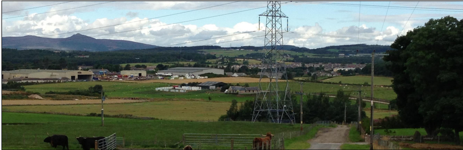
View of site looking north west ( View 3 )
