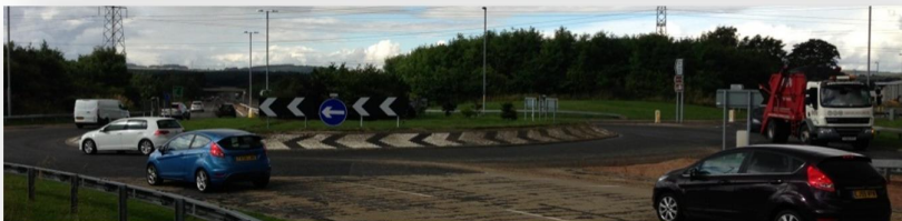
Figure 25 – Broomhill roundabout on A96 trunk road
