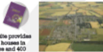
AERIAL VIEW OF SITE
