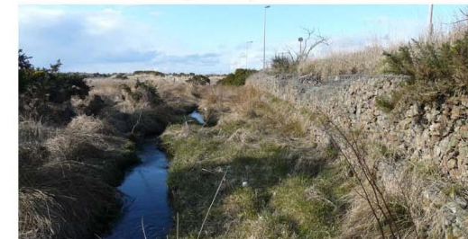
Fig 8. Riparian area view north. Gabion basket supports for Boothby Road can be seen on the right.
