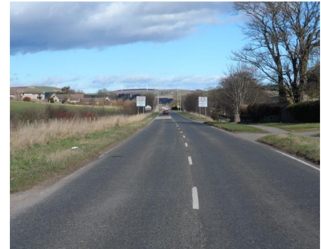
View North along A92 in front of site
