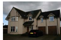
Housing Development on Duthie Road
