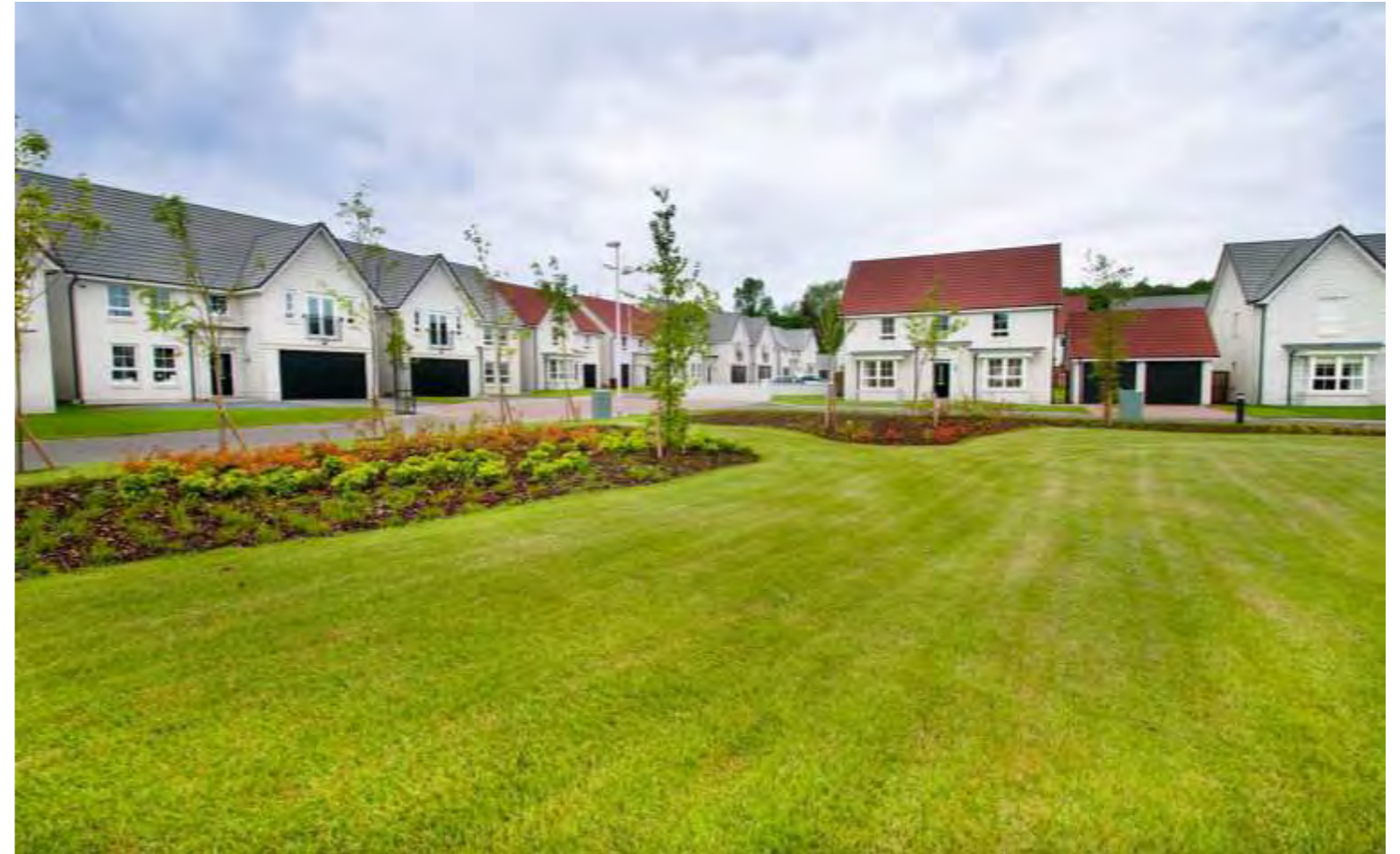
Figure 04 - Barratt North Scotland development at Den of Pitfodels, Aberdeen - completed in 2016
