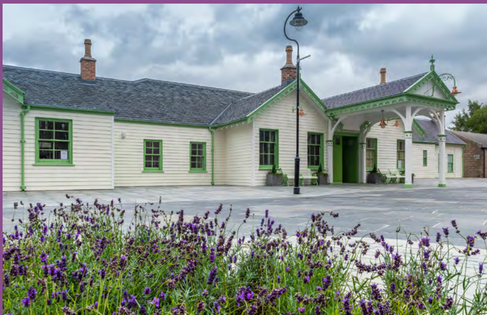
Ballater Station officially re-opened 20 August 2018
