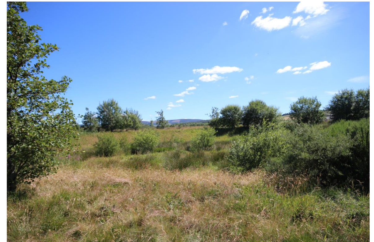
Figure 9 – Existing established SUDs Basin
