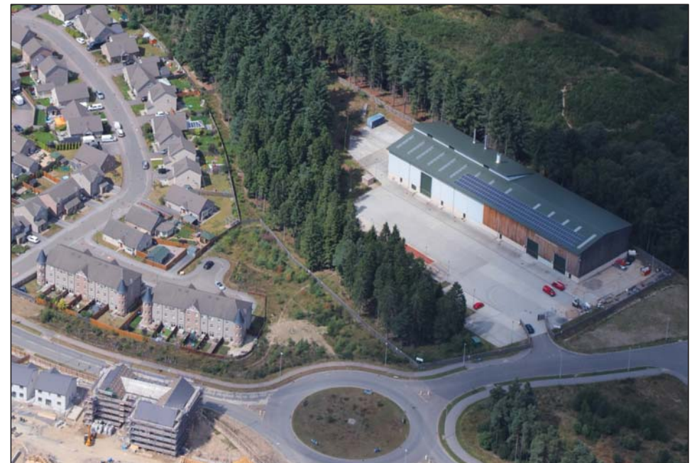
The biomass fuelled energy centre was completed in 2012.
