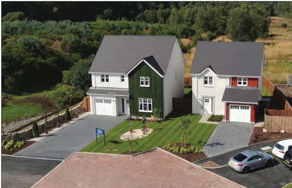
The first two houses in Phase 1a are complete
