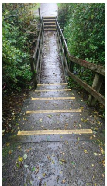
**Management proposals** – The wooden bridges should be inspected regularly and maintained. Broken chicken wire should be removed and an anti-slip coating applied. The steps down to the bridges and path linking these to the Moss should be repaired and maintained.
