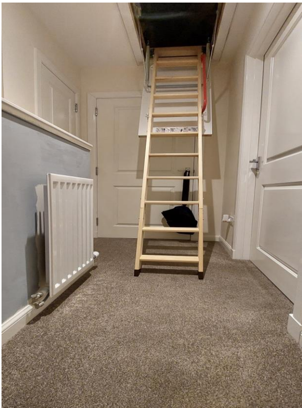
Top Landing with Attic Access
