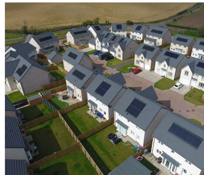
Example of PV panels fitted to roof
