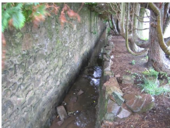
Arbuthnott Drain during Heavy Rainfall
