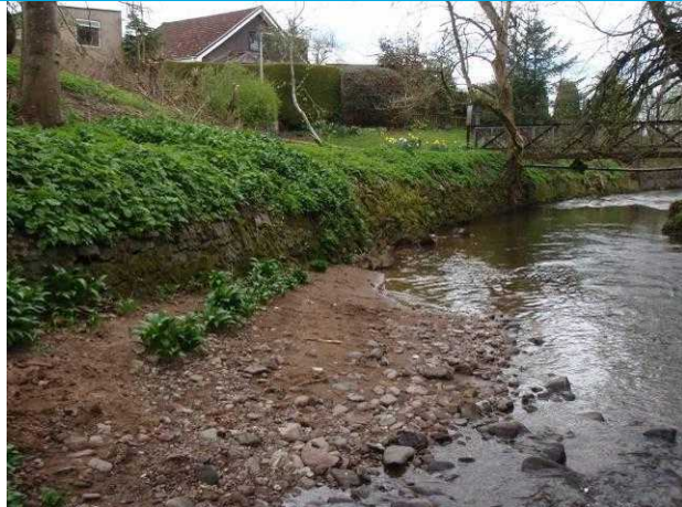
Photograph 3: View of wall on inside of bend some evidence of erosion at base.
