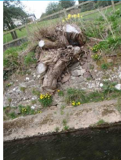
Photograph 10: Close up. Base of wall has been pointed in places with cement based pointing, note loose stones.
