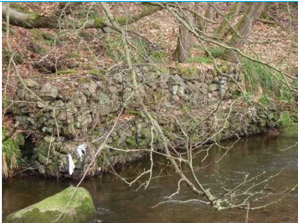
Photograph 1: View of gabion wall, looks like there is a void behind the wall.
