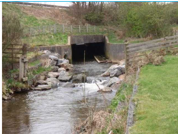
Photograph 3: Gabion Wall on RHB below exit to culvert, wall looks uneven. Note placement of stones in front of wall.
