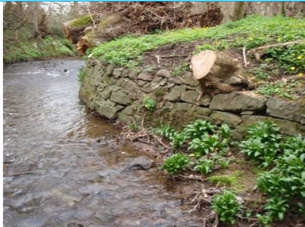
Photograph 3: View of wall on inside of bend some evidence of erosion at base.
