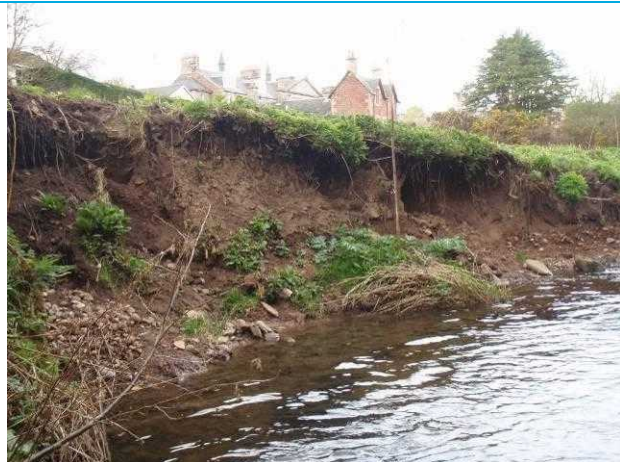
Photograph 1: View showing bank erosion
