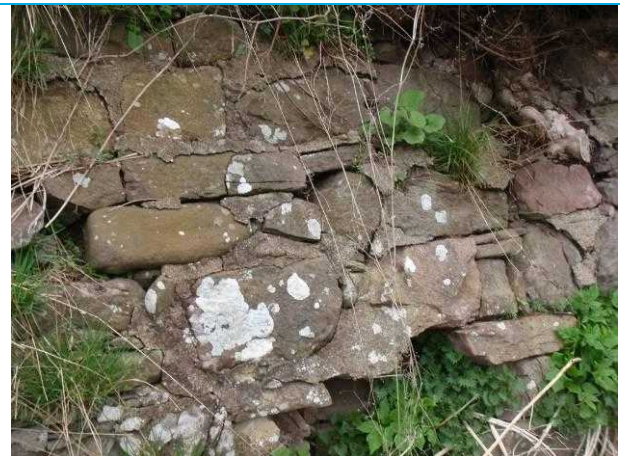
Photograph 10: Close up. Base of wall has been pointed in places with cement based pointing, note loose stones.
