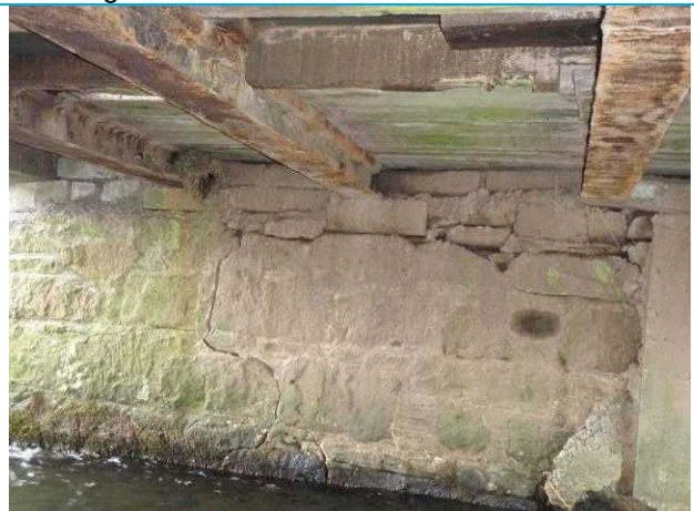
Photograph 2: View of LHB abutment, note cracking and erosion of steel beams.
