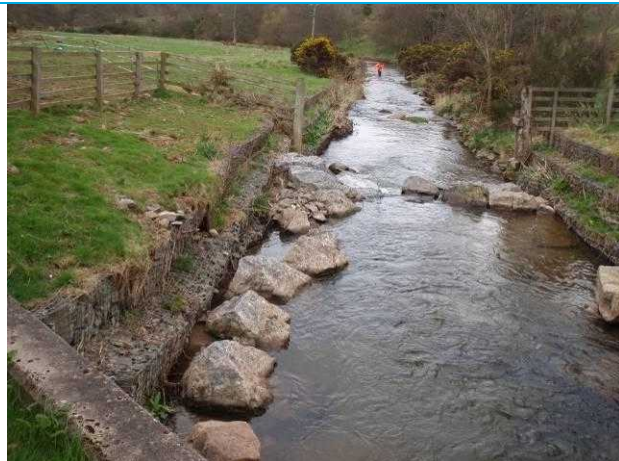
Photograph 3: Gabion Wall on RHB below exit to culvert, wall looks uneven. Note placement of stones in front of wall.
