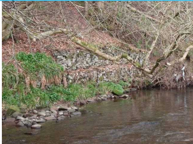
Photograph 1: View of gabion wall, which is well vegetated.
