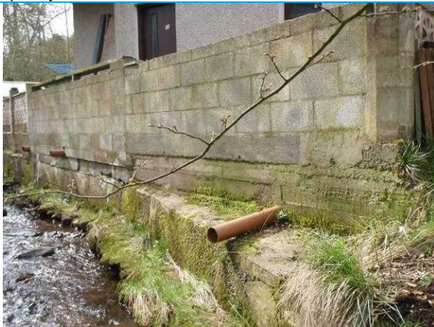
Photograph 3: Note vegetation at base and general poor quality.
