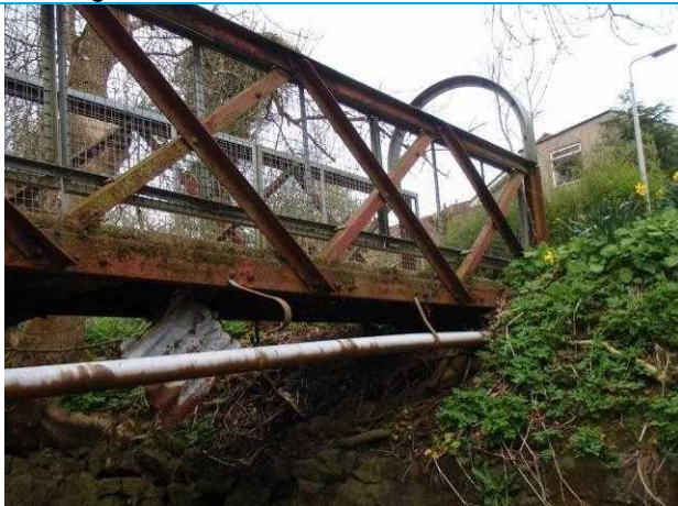
Photograph 3: View showing duct detached from support brackets, and detached corrugated steel decking
