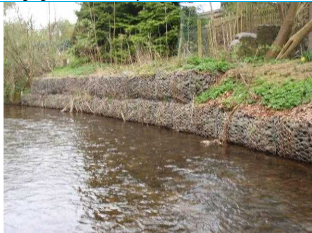
Photograph 1: Gabion wall, showing some signs of bulging, looks relatively recent.
