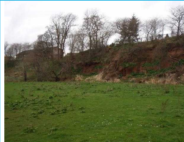
Photograph 1: View of steep bank on outside of bank showing extensive signs of instability.
