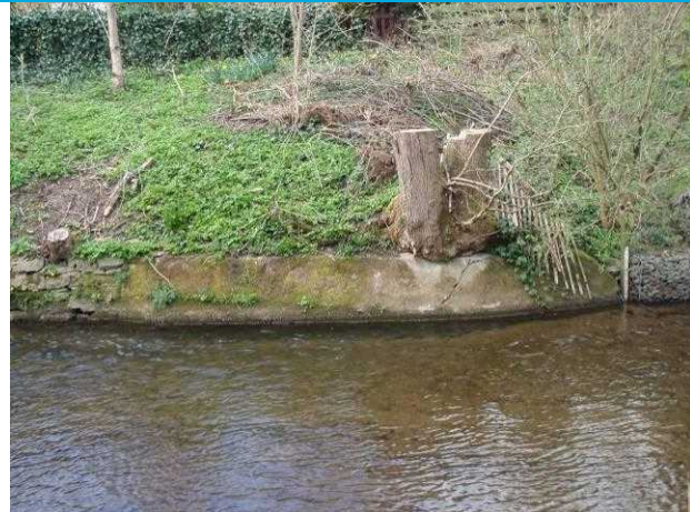
Photograph 1: View of rendered wall showing signs of cracking, and vegetation growth.
