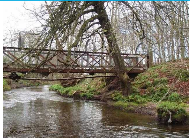
Photograph 4: View showing corrosion of steelwork
