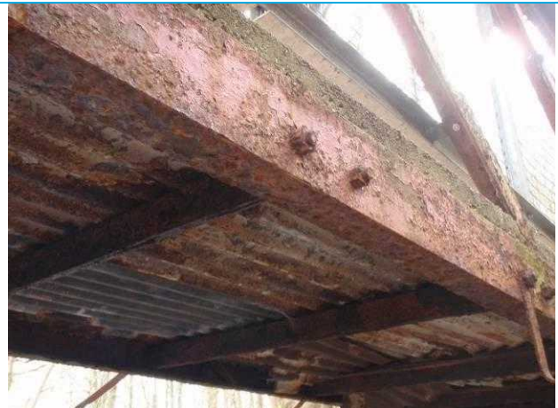
Photograph 4: View showing corrosion of steelwork
