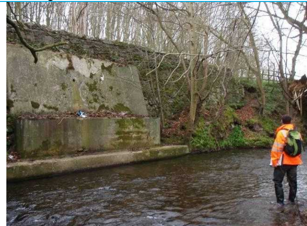
Photograph 2: Middle and upstream end of wall, showing area of loose stonework.
