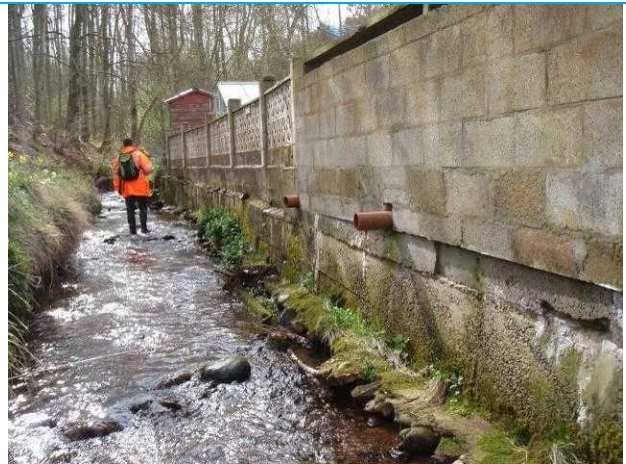
Photograph 2: Note undermining at base
