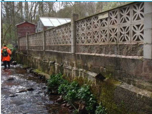
Photograph 3: Note vegetation at base and general poor quality.
