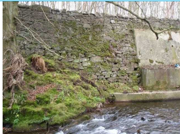
Photograph 1: Downstream end of wall, showing area of loose stonework.
