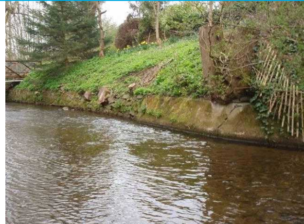
Photograph 2: View of wall up to bridge. Note tree growth.
