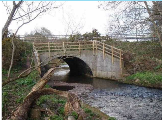
Photograph 3: View of concrete arch culvert looking downstream.
