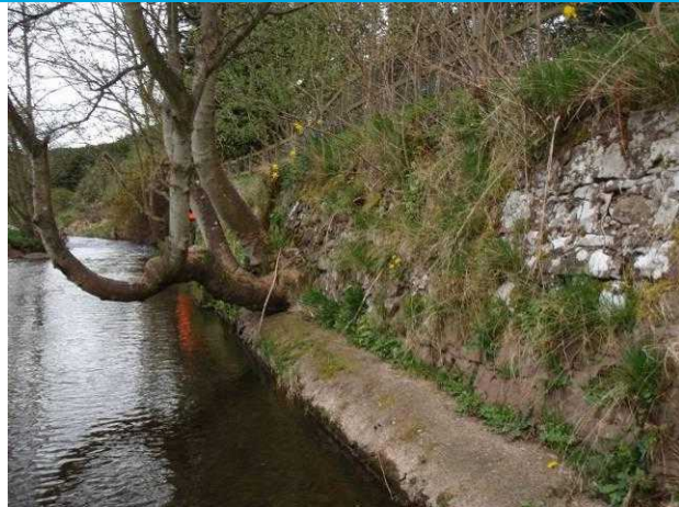
Photograph 11: Tree growth from base of wall (tree has been ring barked).
