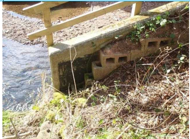
Photograph 4: View behind wing wall, showing possible erosion.
