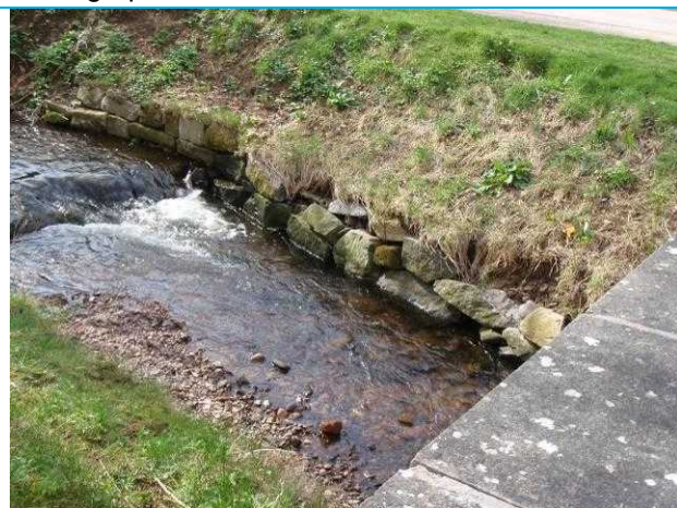
Photograph 1: View of wall.
