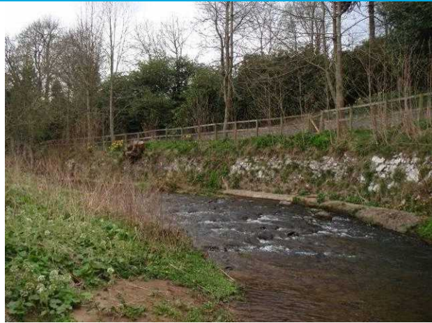
Photograph 7: Drystone wall, note concrete cill.
