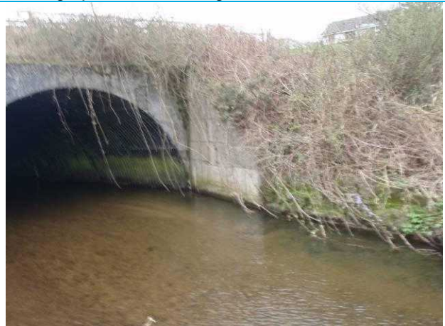
Photograph 4: View behind wing wall, showing possible erosion.
