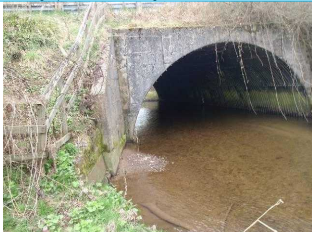
Photograph 3: View of concrete arch culvert looking downstream.
