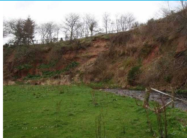
Photograph 2: View of steep bank on outside of bank (cont.).
