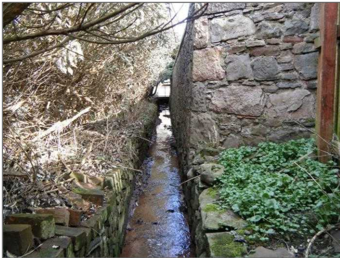
Figure H-0-5: Photograph showing open section of Arbuthnott Drain
