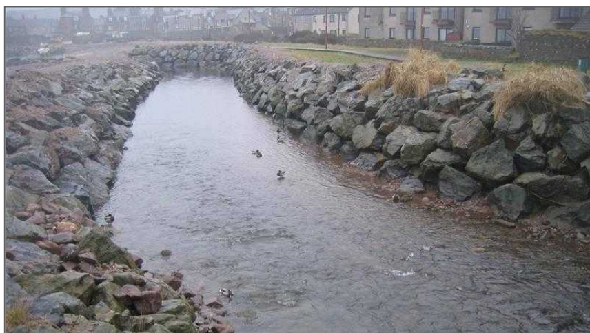
Figure H-0-7: The modified armoured channel of the Carron at the coastal outfall
