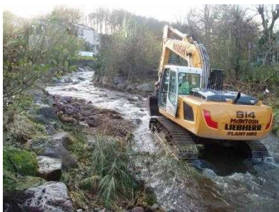
Emergency repairs in 2009
