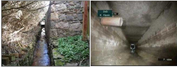
Open section of Arbuthnott Drain Under Arbuthnott Court
