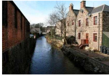
Looking upstream from Bridgefield Bridge
