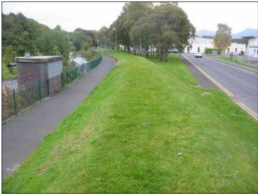
Example Photograph of Flood Defence - Galashiels
