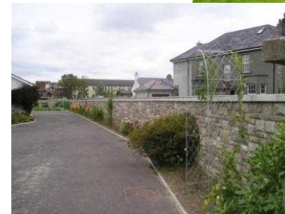
Example Photographs of Flood Walls
