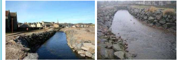
Rock armour along River Carron at its outfall into the North Sea
