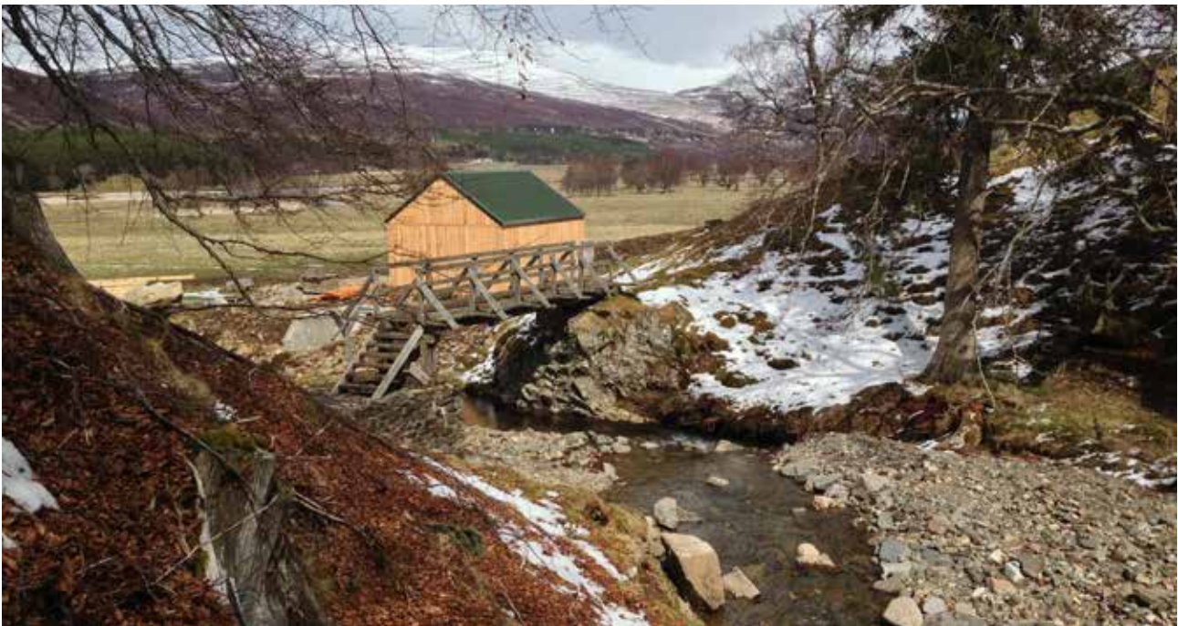
Turbine House at Braemar Community Hydro, Corriemulzie
