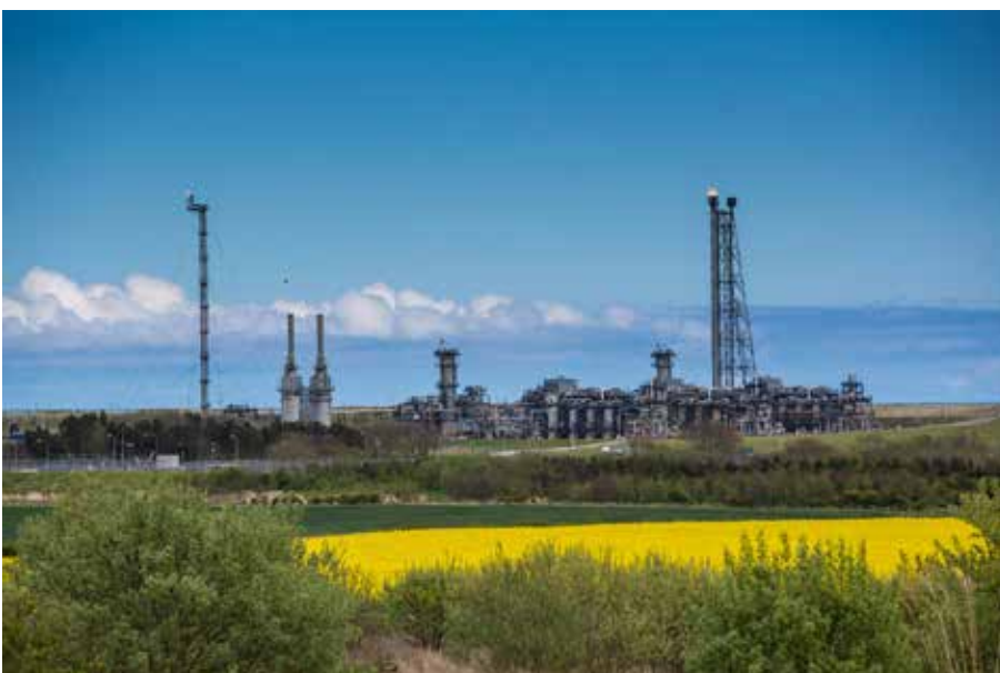
St Fergus Gas Terminal Image courtesy of px Limited
