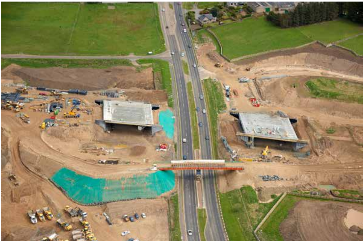
Preparatory work for river and road crossings on the AWPR at Peterculter (top) and on the A944 near Westhill
