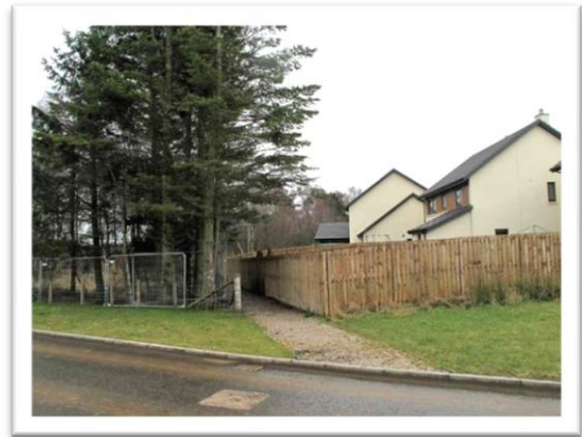
Figure 5 - Entrance 4 between existing houses and construction site. Not a key entrance.
