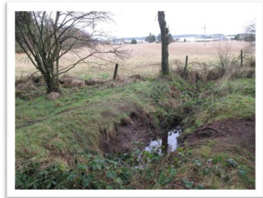
Figure 6 - Culverts will be needed on an all abilities path to cross drains and ditches
