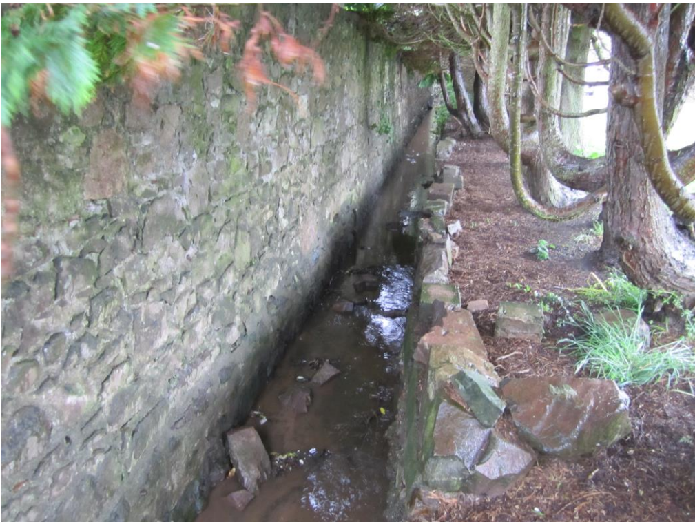
Figure 2-2: Photographs of Existing Mill Lade
