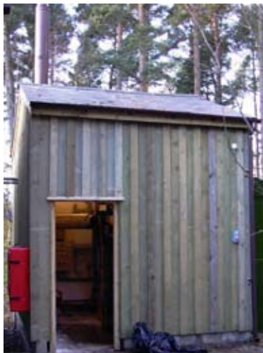
Boiler shed showing the flue (image courtesy of the Forestry Commission)
