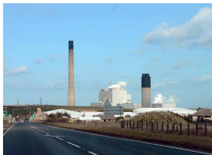
Peterhead Power Station
