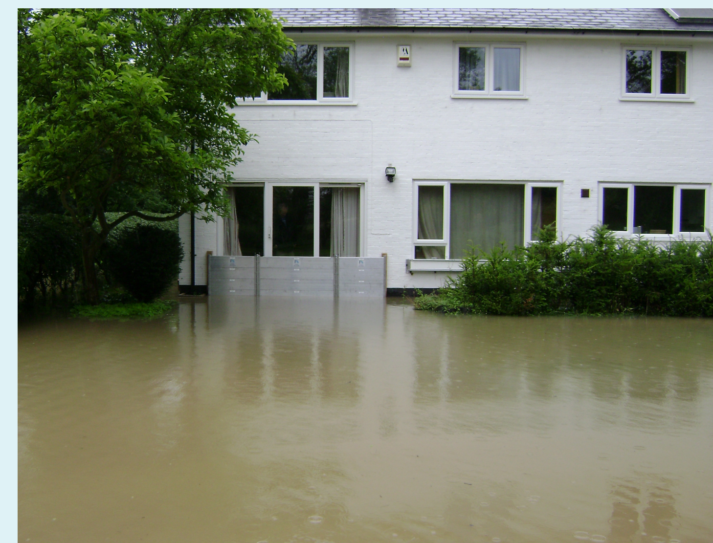
Property Level Protection measures, including [top left, bottom right] door barriers; [top right] temporary barriers, reinforced with sandbags; [below] air brick cover.
