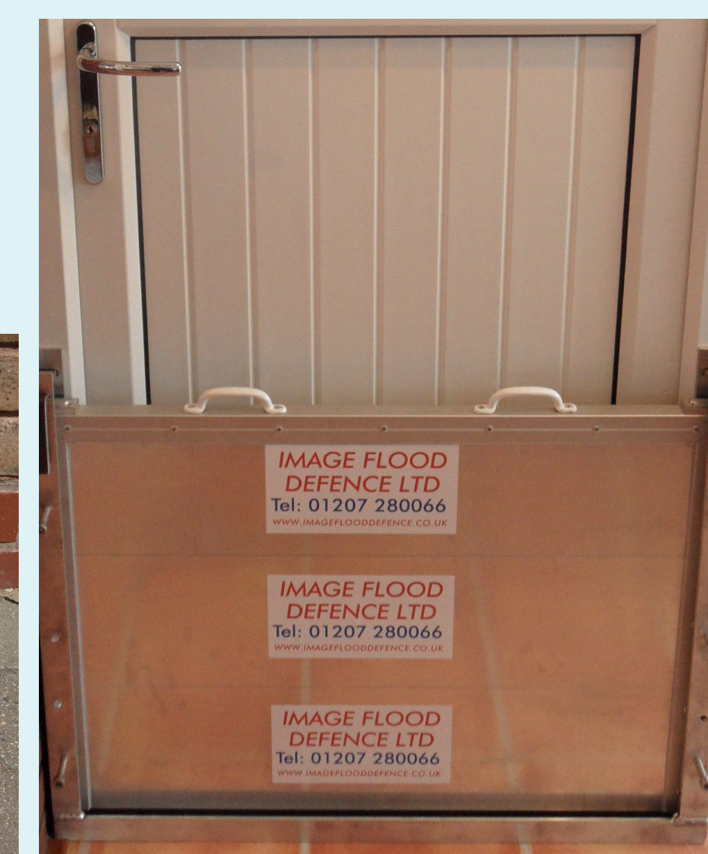
Property Level Protection measures, including [top left, bottom right] door barriers; [top right] temporary barriers, reinforced with sandbags; [below] air brick cover.
