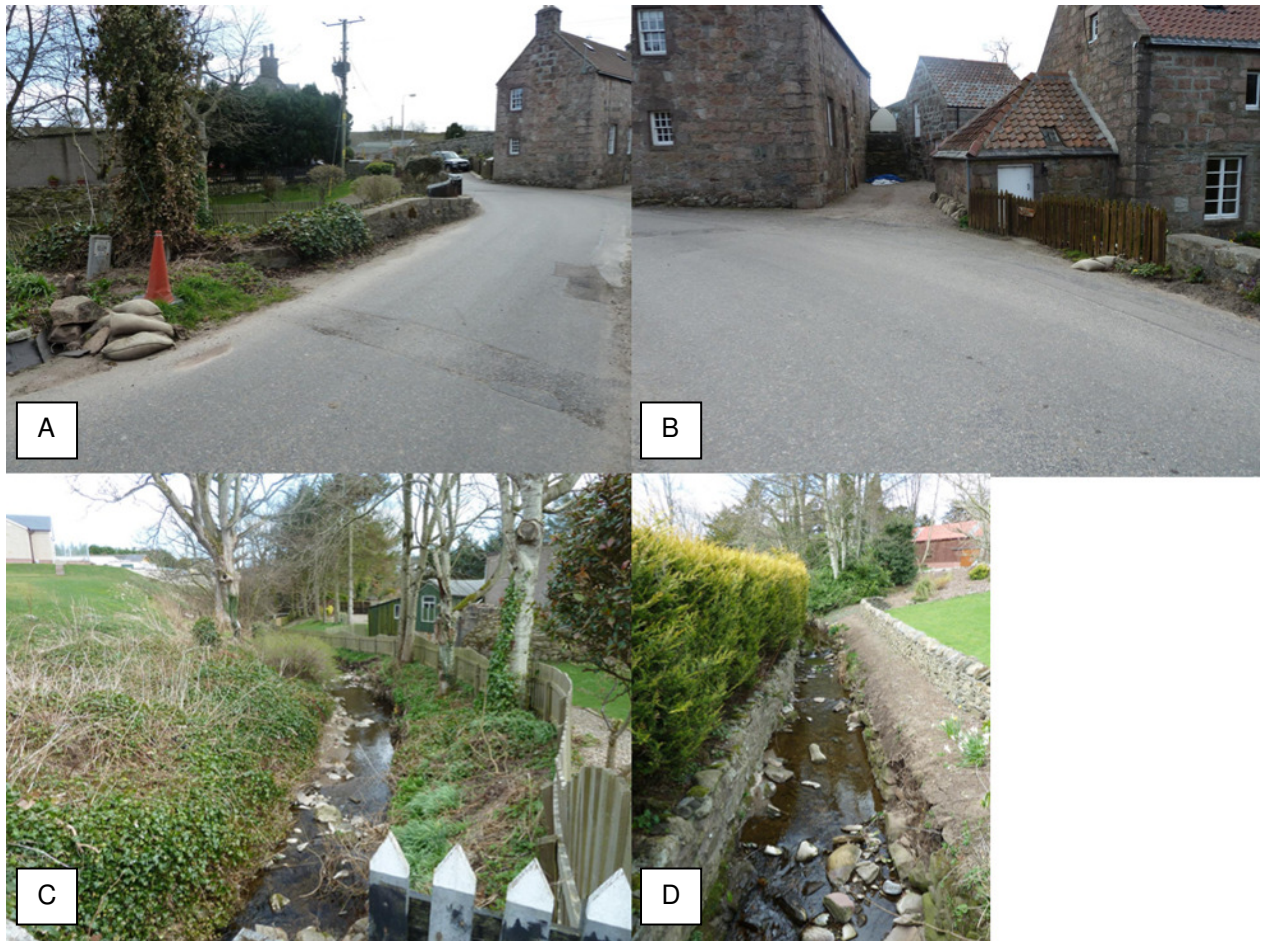
Figure 3-8: Cheyne Burn at Bridge of Fetteresso
