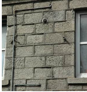
Example of stone erosion caused by cement pointing
