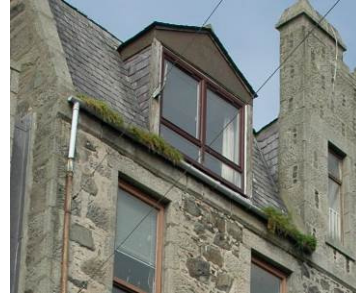
Gutter blocked by weeds and rusted downpipe
