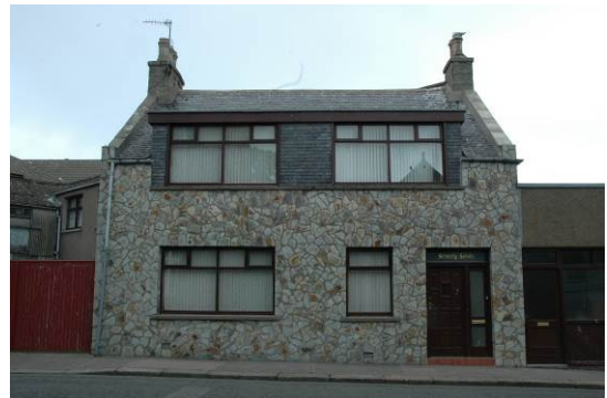
77 Commerce Street, possibly late 19 th century? - the original openings now much enlarged, a large wallhead dormer added and inappropriate 'crazy paving' facing to the elevation
