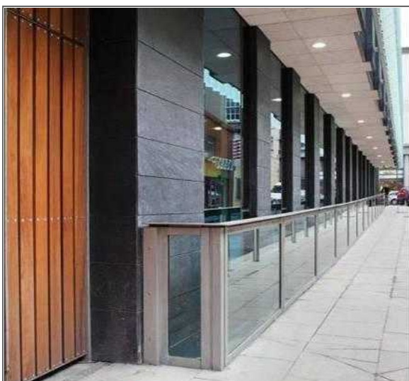
Figure 8-2: Example of glass flood barrier
