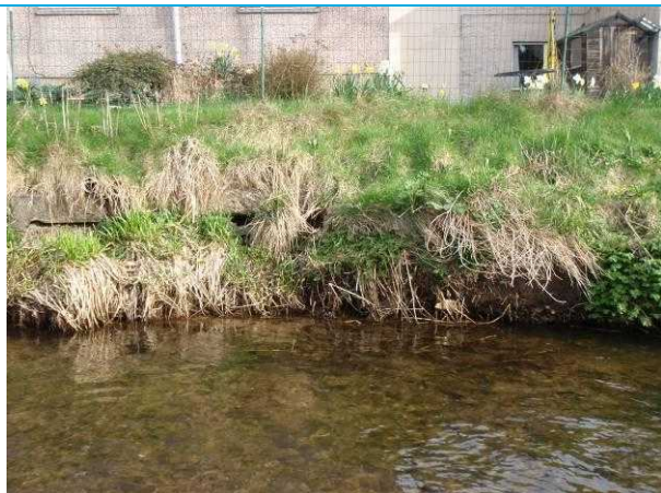
Photograph 3: View of middle of wall, wall possibly partially collapsed and bank vegetated.
