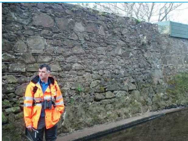
Photograph 3: View of wall showing open joints.
