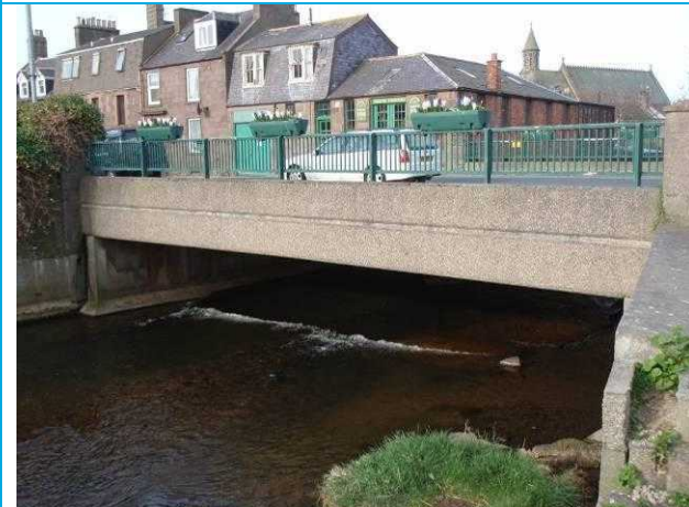
Photograph 3: RHB abutment, note sheet piling to protect toe.
