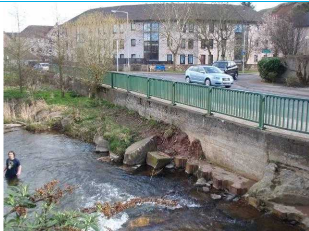
Photograph 3: Spalling to top of concrete wall.
