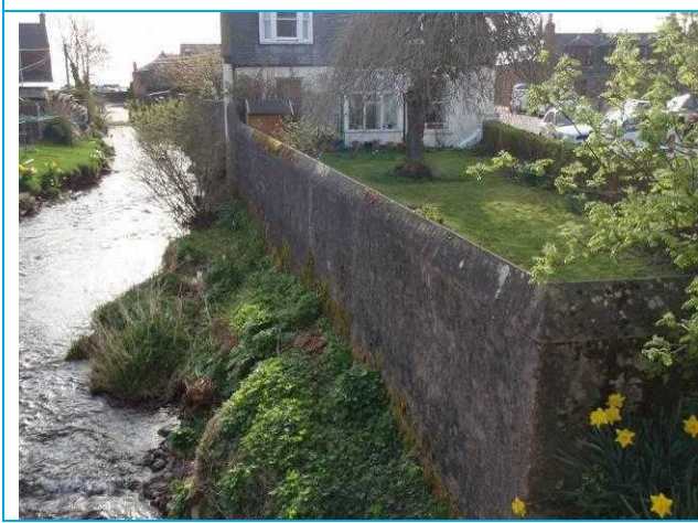
Photograph 5: View looking downstream along wall.
