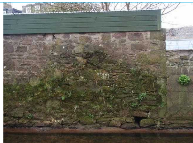
Photograph 4: View of wall showing moss, vegetation and open joints.
