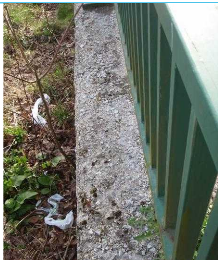
Photograph 3: Spalling to top of concrete wall.
