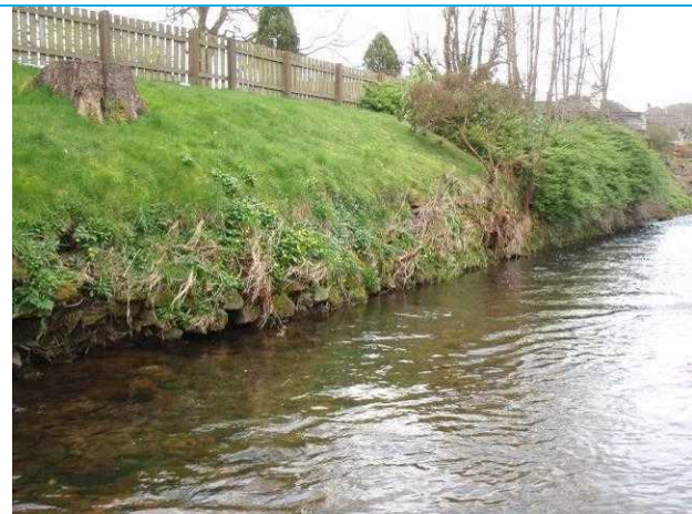
Photograph 4: Dry stone wall at toe of embankment.
