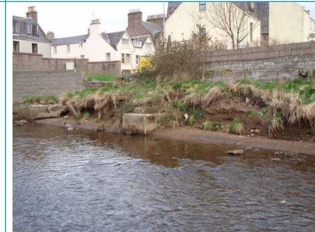
Photograph 4: Upstream end of wall, note erosion at base.
