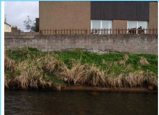
Photograph 3: Note cracking where wall built on older footings.
