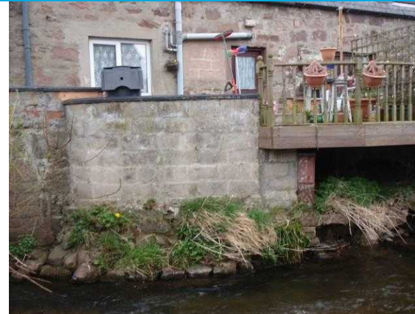
Photograph 4: Blockwork wall upstream of decking.
