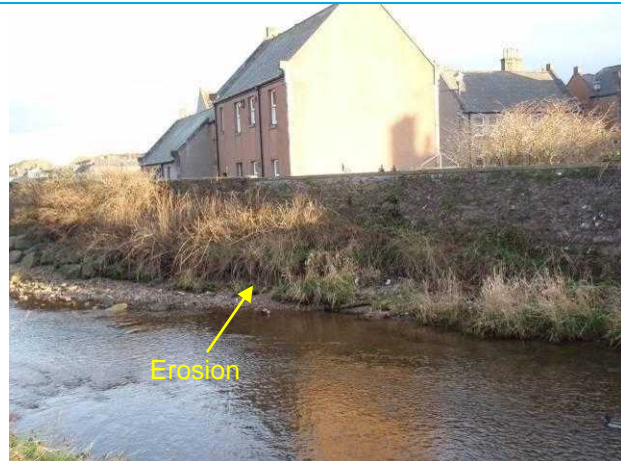
Photograph 3: View of wall looking upstream, note local erosion.
