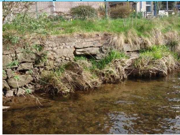
Photograph 4: View of downstream end of wall, wall possibly partially collapsed and bank vegetated.
