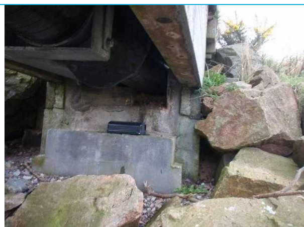
Photograph 3: RHB Abutment, note evidence of previous bridge, below existing beams.
