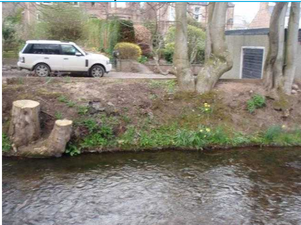
Photograph 3: Earth embankment with mature trees looks relatively stable.
