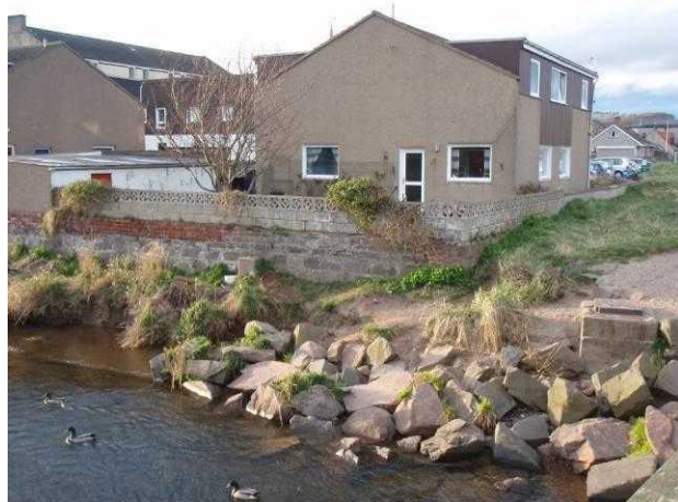
Photograph 1: Single skin masonry wall, on stone wall. Note rock armouring and erosion below.
