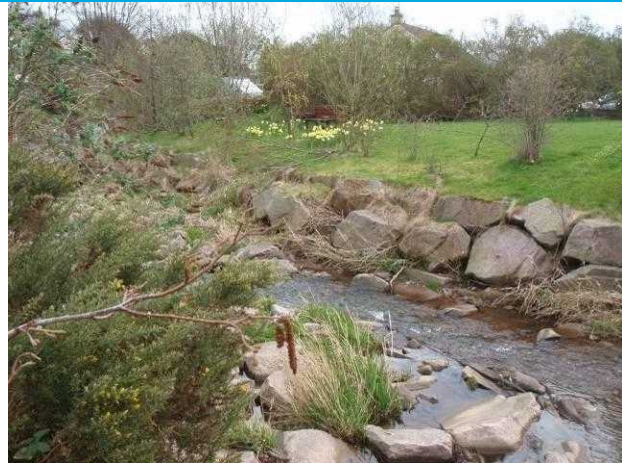
Photograph 12: Rock revetment along fish pass.
