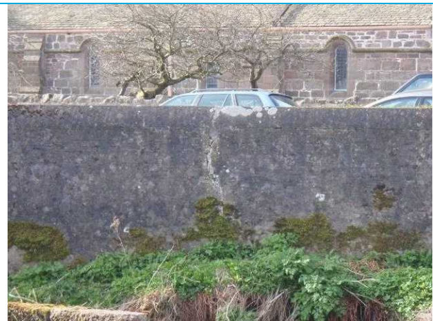
Photograph 4: Crack in wall, likely to be due to thermal and/or moisture movement.
