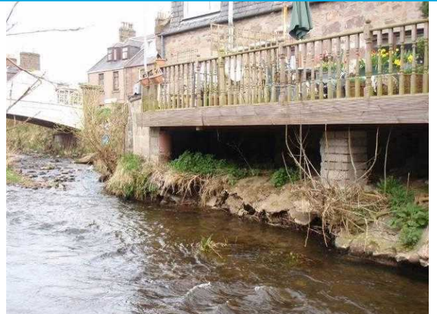
Photograph 3: Foundations to pier supporting decking being undermined.
