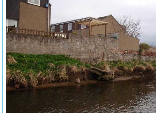
Photograph 4: Upstream end of wall, note erosion at base.
