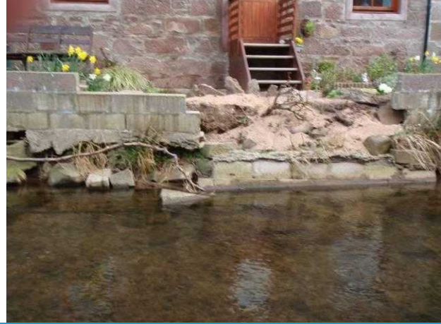
Photograph 3: Upstream end of wall showing collapse of section (believed to have occurred during November 2009 flood event).
