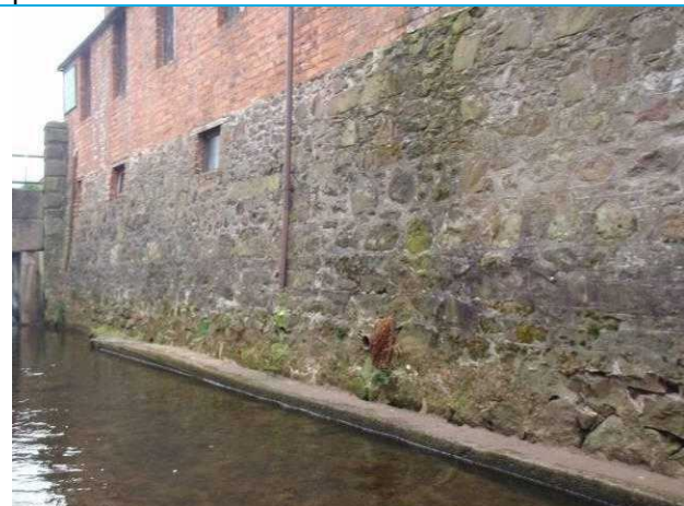
Photograph 4: View of wall showing moss, vegetation and open joints.
