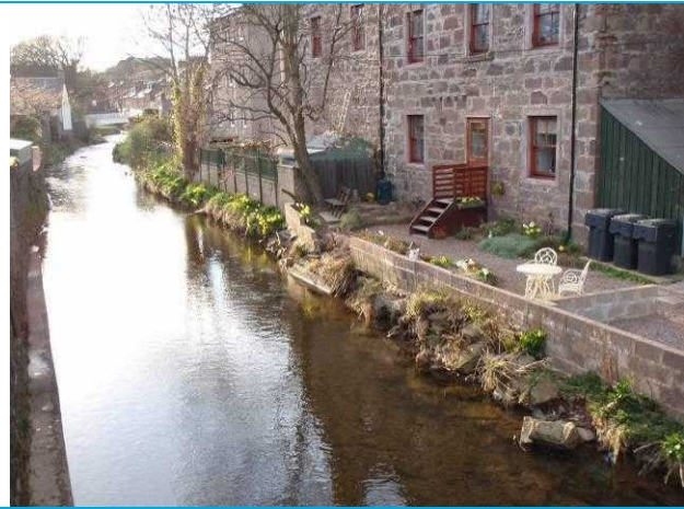
Photograph 3: Upstream end of wall showing collapse of section (believed to have occurred during November 2009 flood event).
