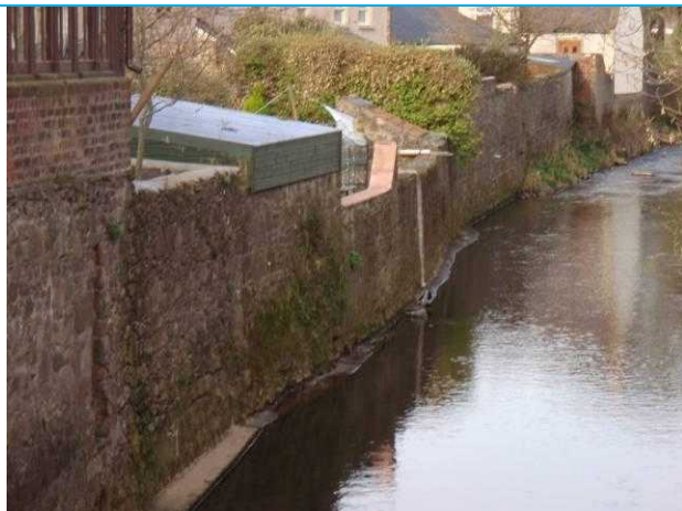
Photograph 3: View of wall showing open joints.
