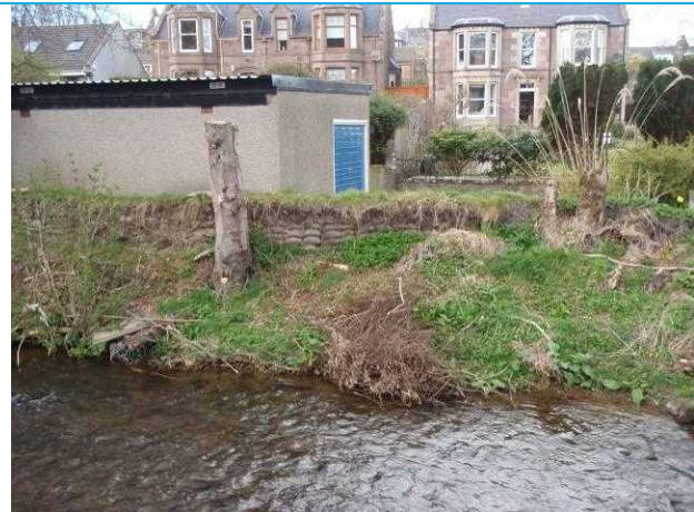
Photograph 4: Sandbag walls around garage.
