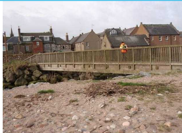
Photograph 3: RHB Abutment, note evidence of previous bridge, below existing beams.
