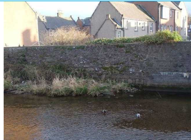
Photograph 4: Western end of wall, note local erosion.
