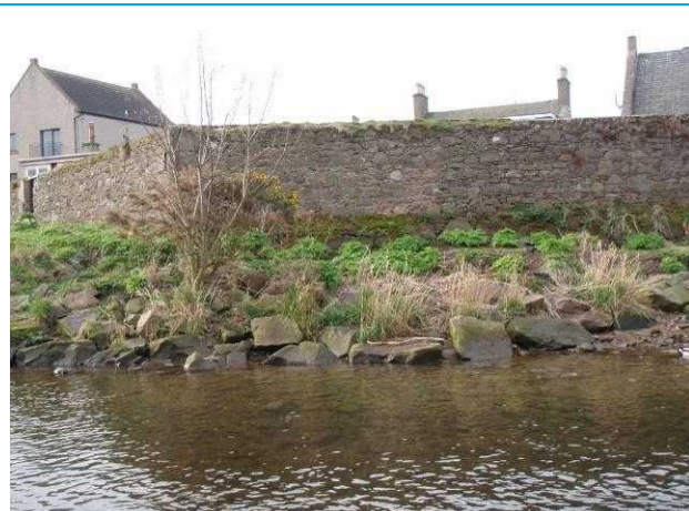
Photograph 3: View of wall looking upstream, note local erosion.
