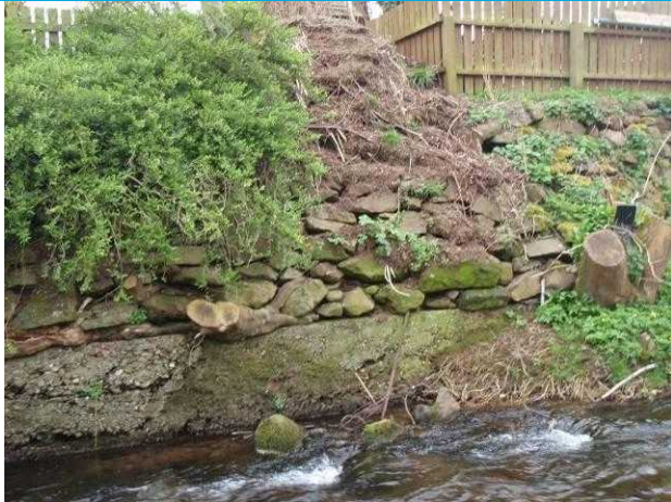
Photograph 7: Dry stone wall built up on embankment.
