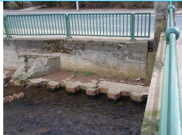
Photograph 2: Sheet pile protection.
