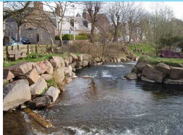
Photograph 2: Boulder walls to sides of weir.
