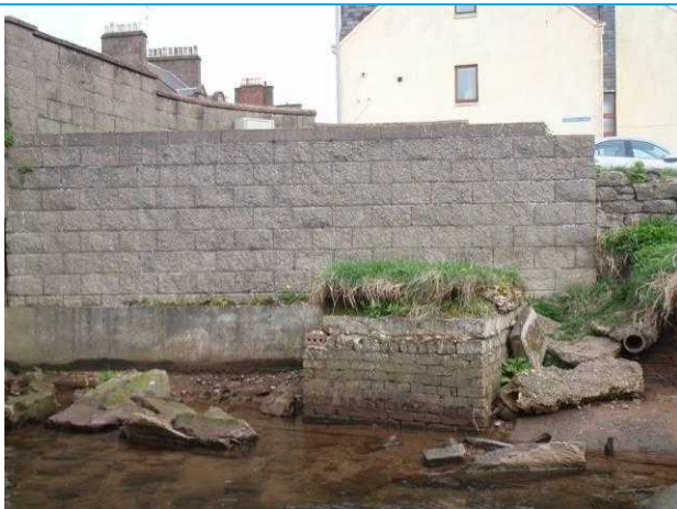
Photograph 1: View of wall and chamber.
