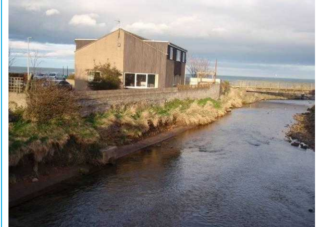
Photograph 3: Note cracking where wall built on older footings.
