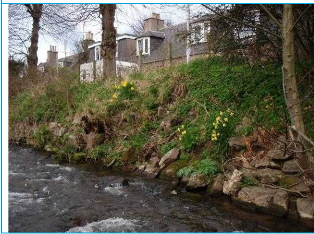
Photograph 5: Vegetated stone bank showing signs of past erosion.
