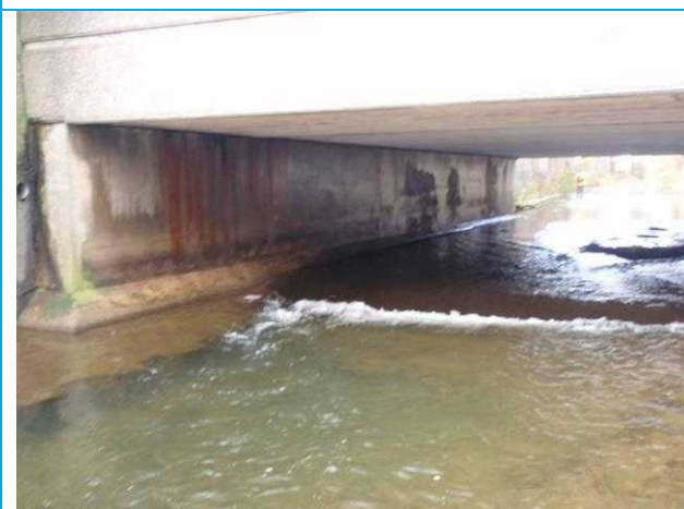
Photograph 3: RHB abutment, note sheet piling to protect toe.
