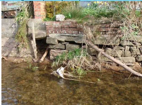
Photograph 3: View of middle of wall, wall possibly partially collapsed and bank vegetated.
