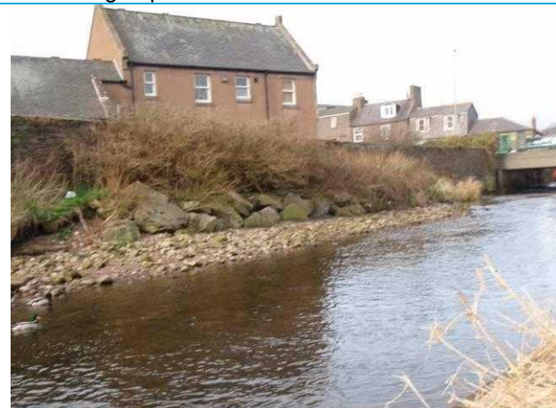
Photograph 4: Western end of wall, note local erosion.
