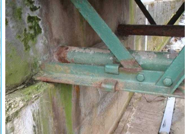
Photograph 4: Beam bearing LHB.
