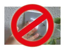
The standard electrical sockets in the UK are so designed that is not possible for a baby or small child to put their fingers into a 13 Amp socket. Until the earth pin of a plug (or of a socket cover!) is inserted, the live parts of the socket are shuttered and protected.
