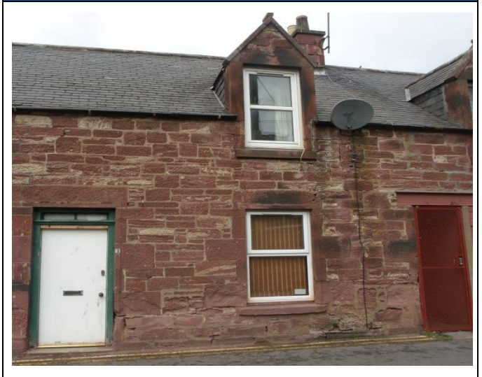
View of the front of house
