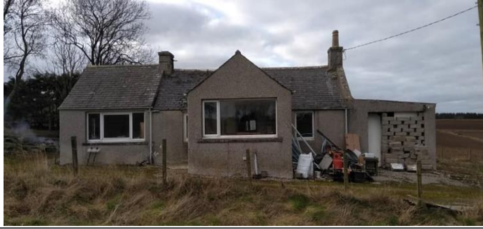
View from the front of house
