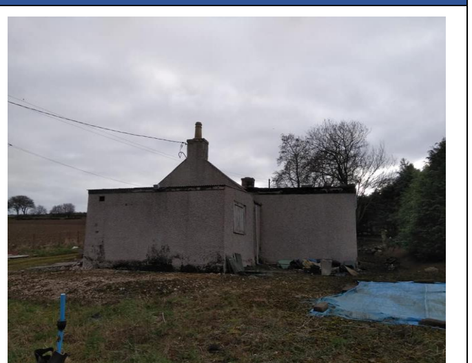
Side view of house and garden area
