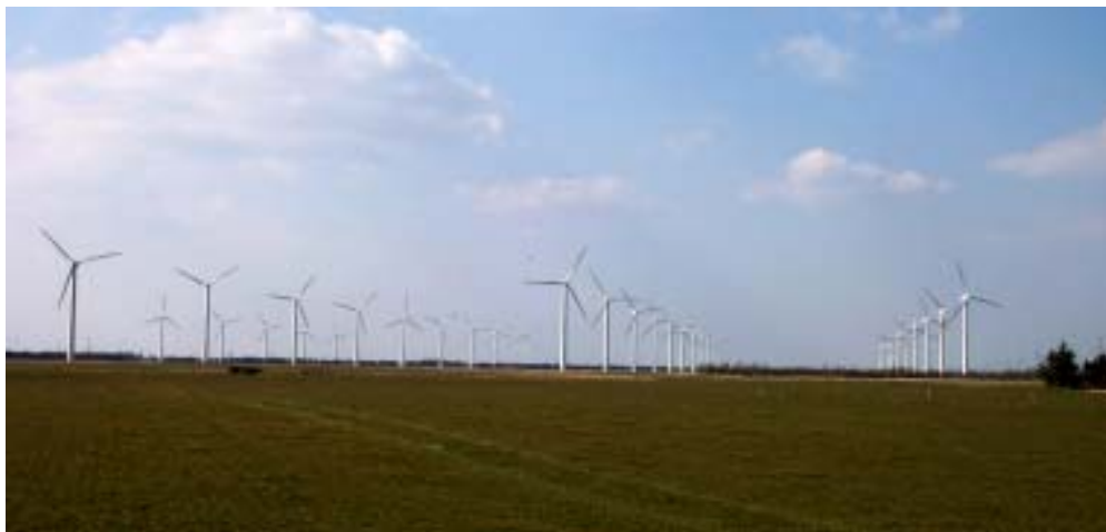
Fig.6 Turbine farm featuring parallel row layout, designed to minimise visual clutter
