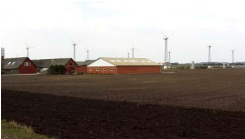
Fig.9 Example of poor turbine planning practice in terms of turbine design and location
