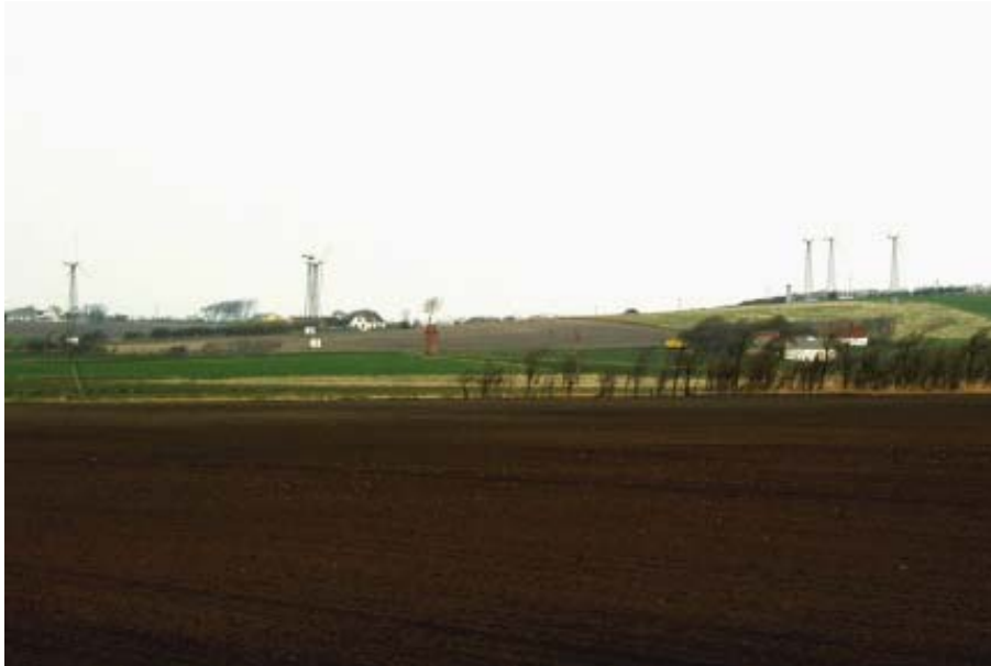
Fig. 19 Example of poor layout and detailing of turbines. These turbines fall under policy to relocate and replace.
