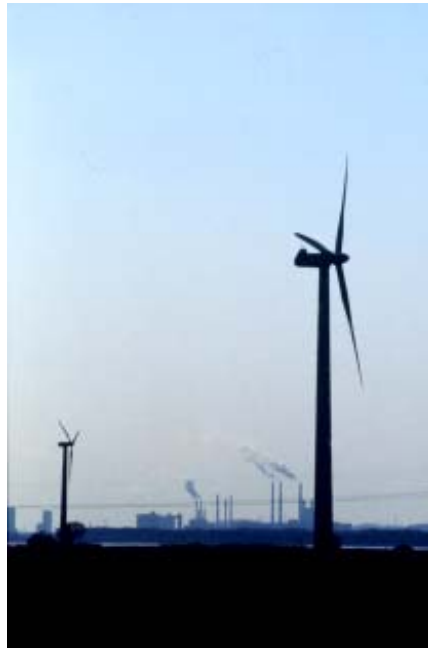
Fig. 10 Turbines located close to Aalborg harbour industrial area
