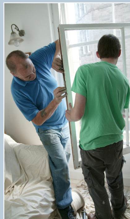
Repairing the sash cords of a timber sash and case window. Most components of a traditional window can be repaired without the waste of replacing the whole unit.
