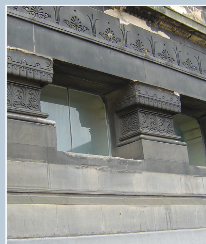
St Vincent Street Church by Alexander 'Greek' Thomson, St Vincent Street, Glasgow. Thomson's Graeco-Egyptian designs emphasised the solid monumentality of the masonry against the void of the window openings. He used large sheets of plate glass and minimal frames to achieve this effect. © S. Dibdin.
