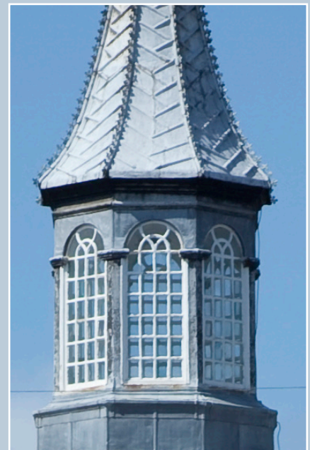
Fixed small-pane windows in the cupola of Robert Gordon's Hospital, Aberdeen, designed by William Adam in 1731–32. Thick astragals (glazing bars) and small panes of glass are typical of this period of design. © N. Haynes.
