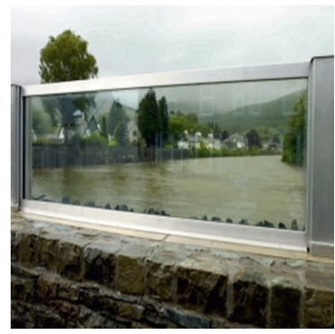
Once the flood water recedes, the water in the reservoir flows from the outlet pipe allowing the self closing barrier to return to its default position
