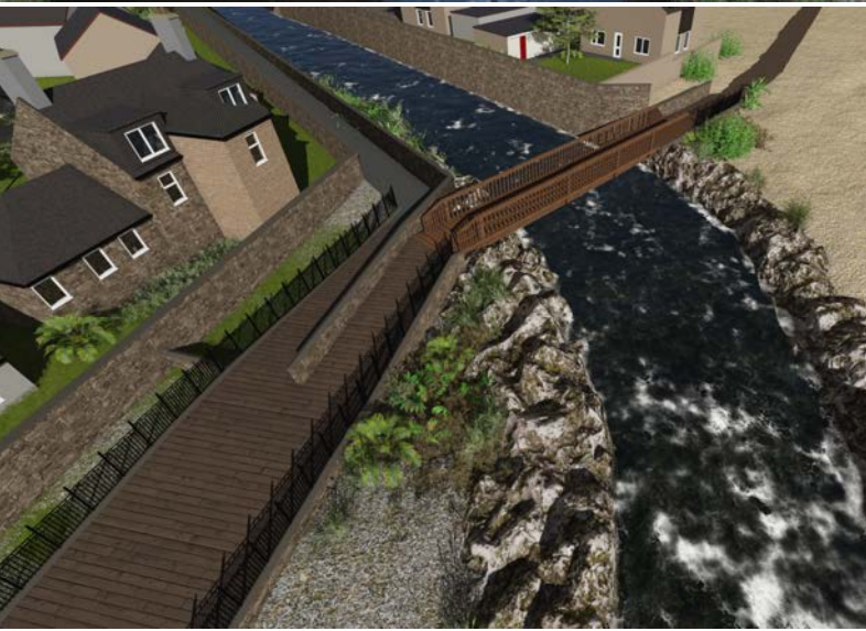
Proposed flood defence solution looking west from Bridgefield. View is indicative of walls without self-raising barrier in operation.
