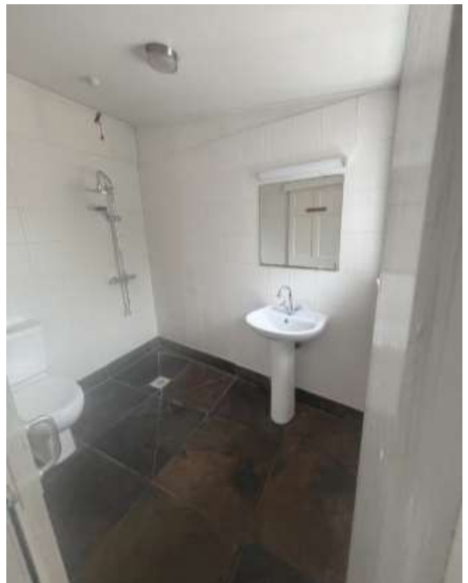
Shower Room (GF)
