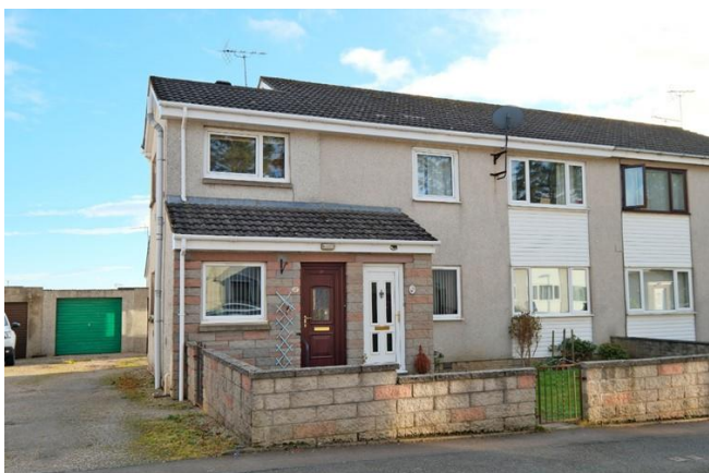
Front of Property
