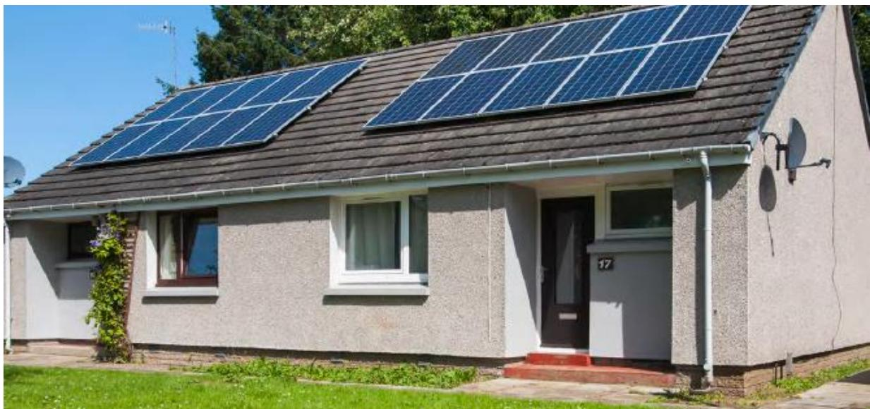
Solar PV can still generate some electricity on cloudy days but does not generate any electricity at night. Not all roof surfaces are suitable for the installation of Solar PV as not enough electricity is generated if the panels don't face due south or they are not on a pitched roof at 35 - 40°. Shading of the panels by other building or trees will also reduce efficiency.
